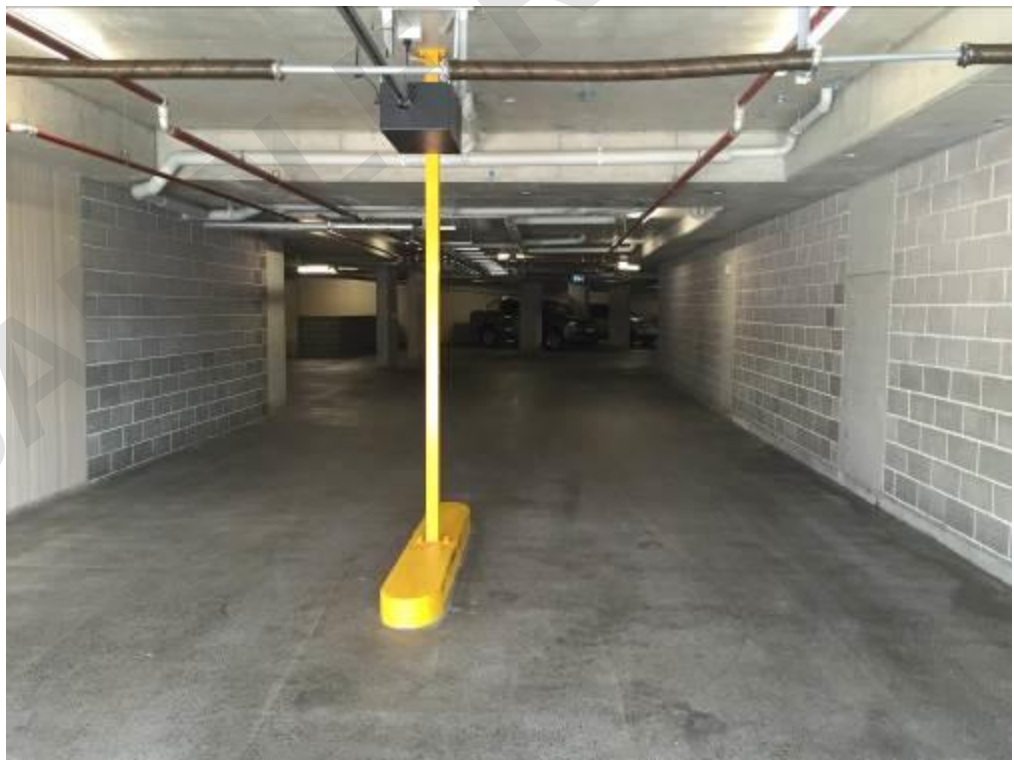
(Car park entry)
