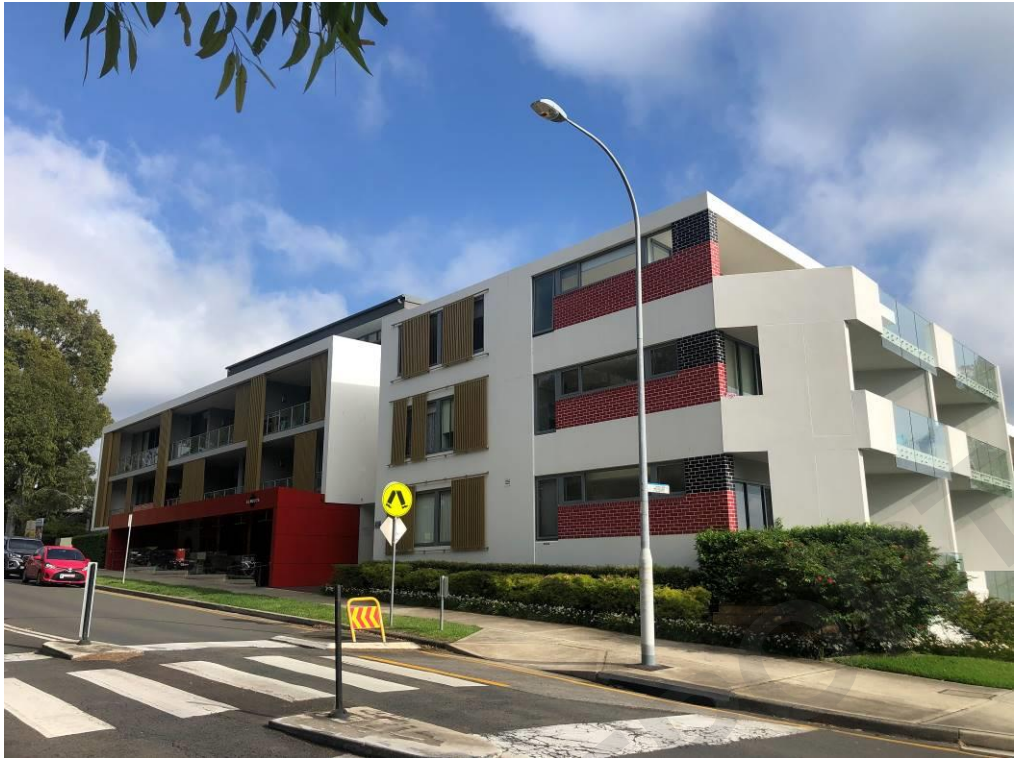
(View of Subject Building)
