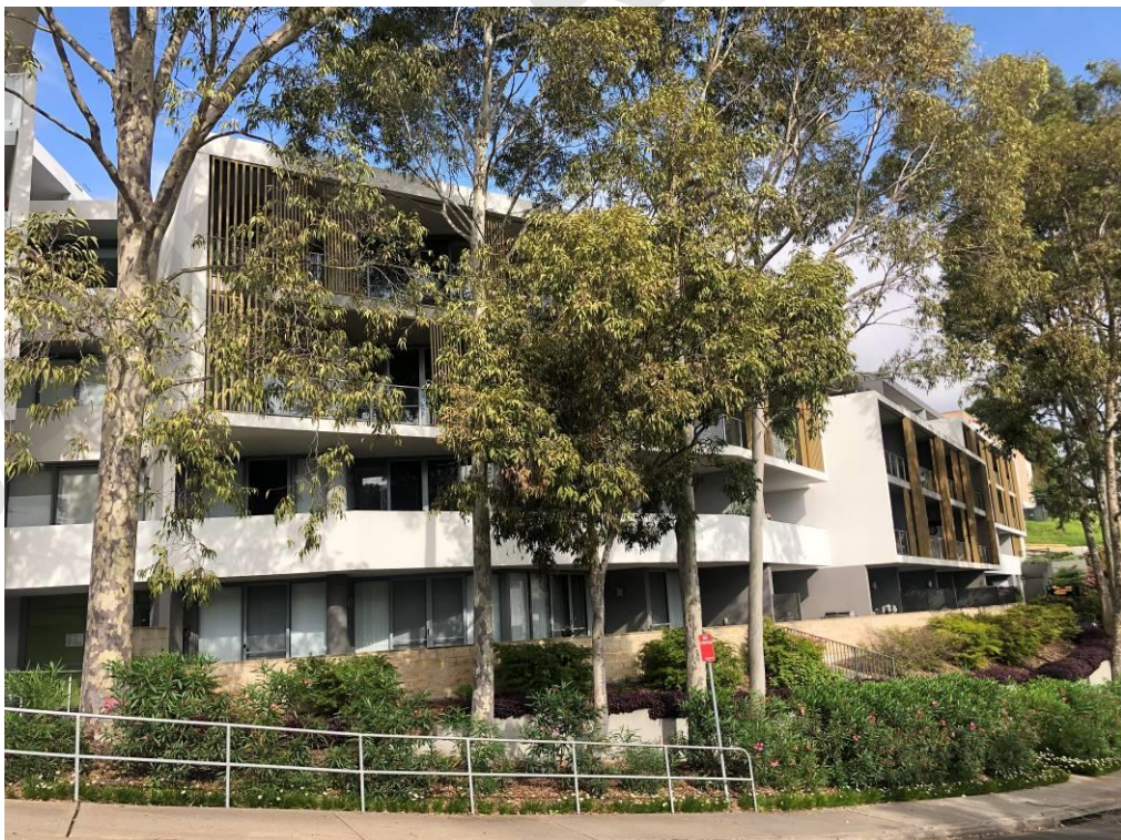
(View of Subject Building)
