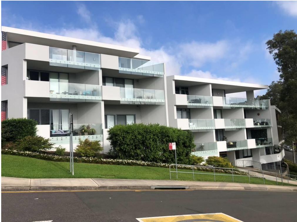
(View of Subject Building)
