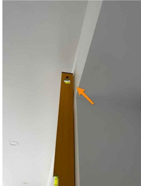
Bow in plasterboard between wall and bulkhead in the kitchen is 4mm
