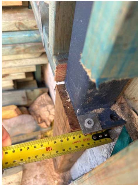
20mm overhang with only a single fixing
