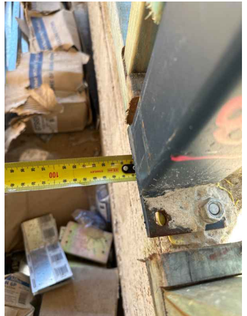
45mm overhang from concrete slab with no fixings into the concrete slab
