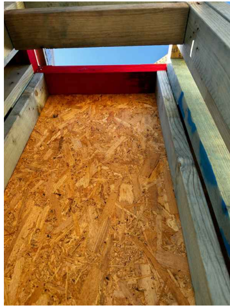
Terminates to the ply bracing
