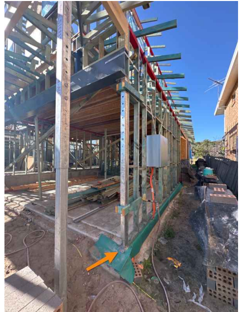
20mm overhang with only a single fixing
