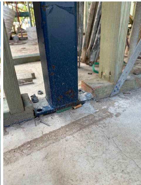
Structural grout and addition bolts require
