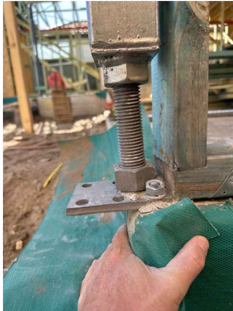
45mm overhang from concrete slab with no fixings into the concrete slab
