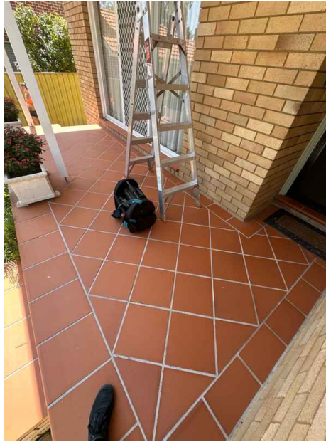
Verandah: General view of Verandah
