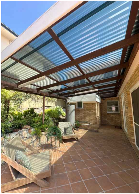
Pergola: General view of pergola
